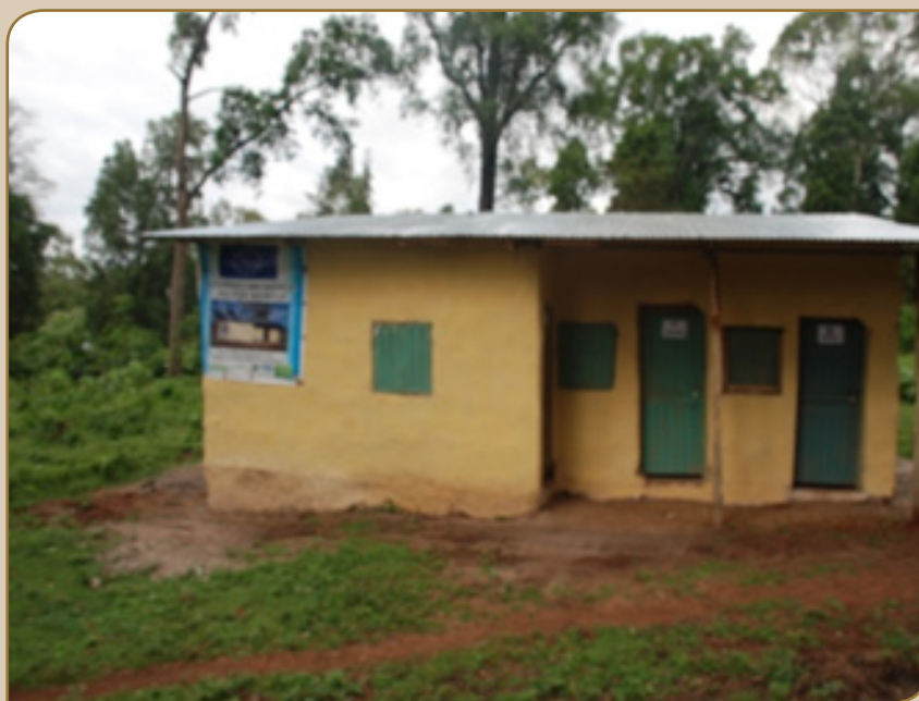
One of the constructed CBO offices
